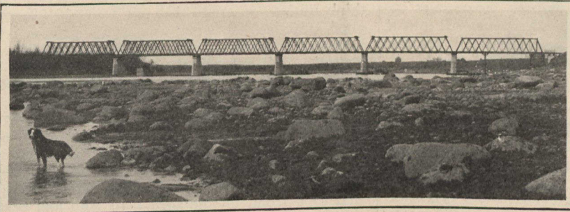
Canadian Northern Railway Bridge.
