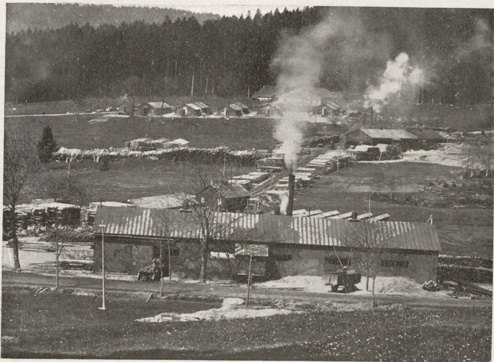
28th Company's Camp in the Vosges Mountains. These mills were designed to cut 20 thousand board feet in 10 hours, but under stress of war average 35 thousand feet, with some record cuts of over 50 thousand feet per ten hours.
