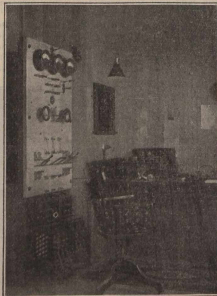
Receiving Apparatus and Switchboard at Sault Ste. Marie.
