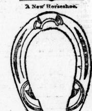
Here is a new idea in horseshoes. It is a shoe fastened to the hoof in the ordinary way, but provided to receive calks that can be removed and replaced by new ones when worn. This can be done by any ordinary stable hand. Each set of these shoes sold is accompanied by twelve dozen calks, which, it is said, will outwear three sets of ordinary
