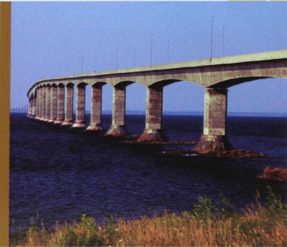
The Confederation bridge links the Canadian provinces of New Brunswick and Prince Edward Island. At 12.9 kilometres, it is the world's longest bridge over ice-covered water. It has won dozens of international engineering awards since its construction, and was designed to last for a century.
