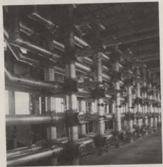
Antenna switching matrix for transmitters at RCI's plant in Sackville, New Brunswick.
