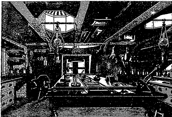
NATURALISTS' WORK-ROOM ON BOARD THE "CHALLENGER."
