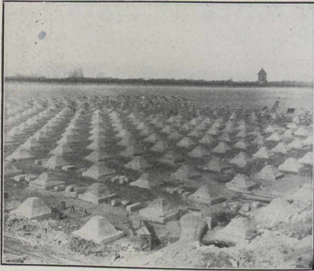
Forms Removed from Pedestal Bases in Clear Water Reservoir.
