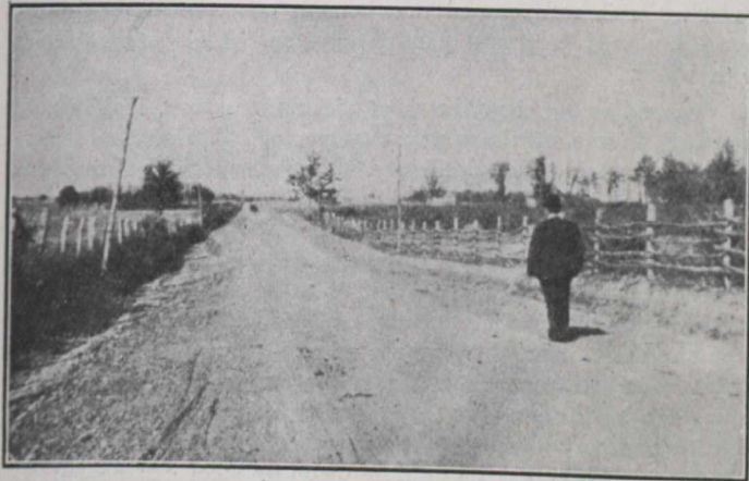
Macadam Object Lesson Road Built in 1904 by United States Office Public Roads, Near Lebanon, Mo.
