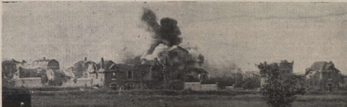
SHELL BURSTING ON THE OUTSKIRTS OF LENS. Canadian Official Photograph.
