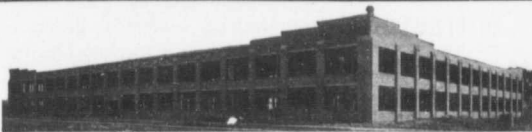
Portion of Plant of A. J. King Piano Co., Bluffton, Ind. Built with Ideal Concrete Machinery.
