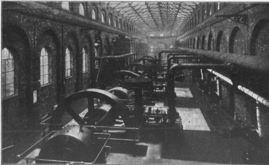
200 H.P. "Premier" Gas Engines and D. C. Generators SOLE CANADIAN LICENSEES
