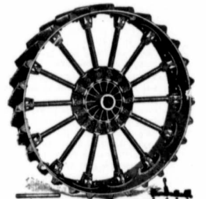
Fig. 197. Wheel used on Gear Steam Traction Engine.
