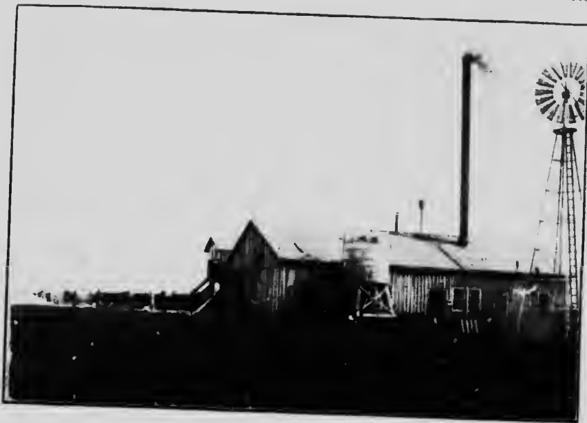
A. Mine building, Crown Gypsum Company, York, Ont.
