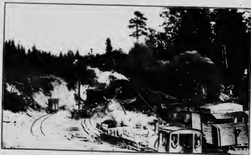
B. Steam shovel at work stripping, Newport Plaster Mining and Manufacturing Company's quarry, Avondale, N.S.
