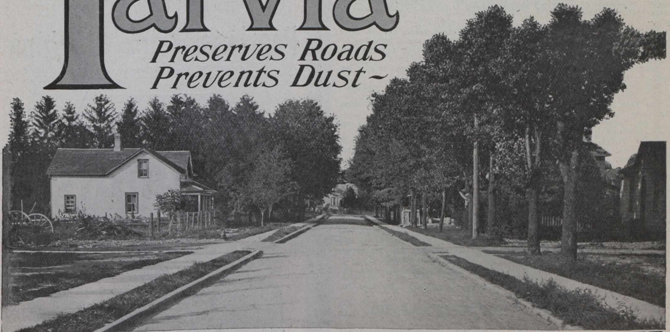
Charles St., Stratford, Ont., showing modern pavement constructed with "Tarvia X"
