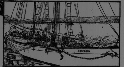
When Captain MacMillan originally equipped "The Bowdoin" for her voyages to the Arctic Regions he chose as his power plant a 45 h.p. Fairbanks-Morse "C.O." Engine. This engine was put to very severe tests and was found to be perfectly reliable under every condition. It was even found to operate perfectly on whale oil.
