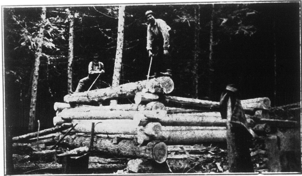
BUILDING A RANGER'S CABIN IN BRITISH COLUMBIA.
