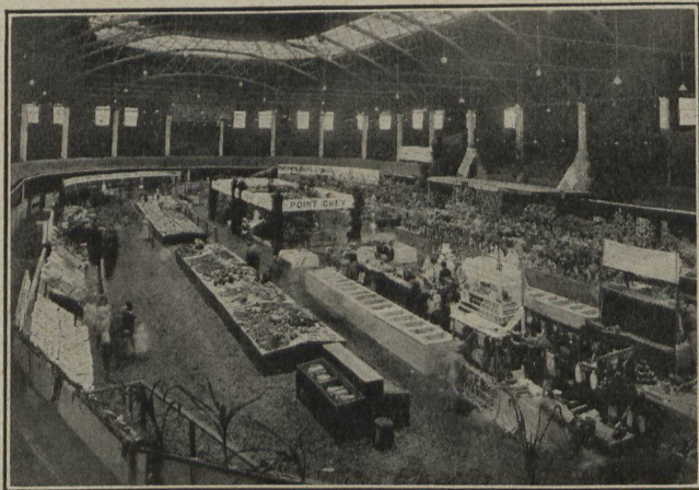
General View Interior Agricultural Buildings, Vancouver Exhibition, 1916.
