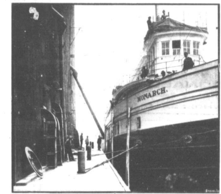
Vessel Loading Wharf
