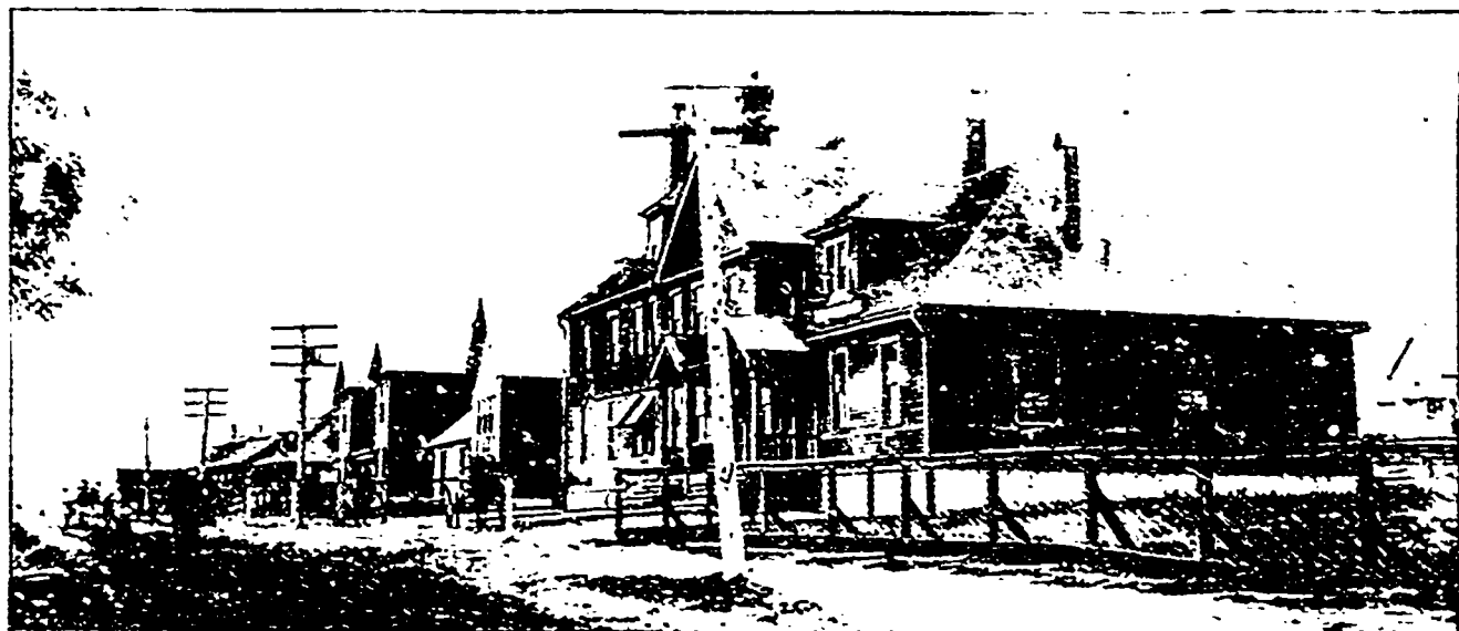
GENERAL OFFICES AND LABORATORY OF THE DOMINION COAL CO., GLACE BAY, C.B.
