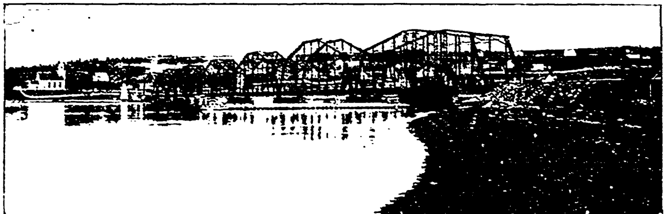
I.C.R. RAILROAD BRIDGE AT GRAND NARROWS, C.B.
