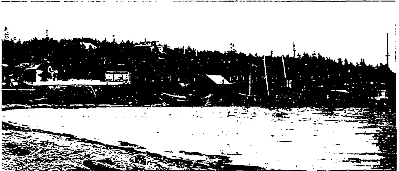
BURCHELL BROS COAL SHIPPING PIER, NEW CAMPBELLTON, C.B.
