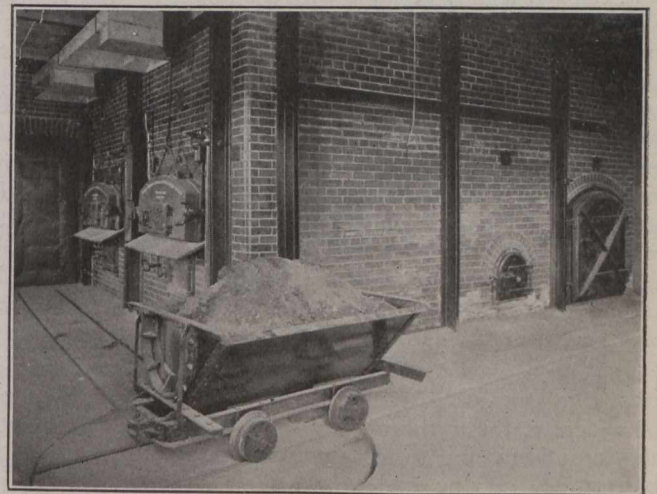
Fig. 3.—Clinkering Doors and Type of Car Used.
