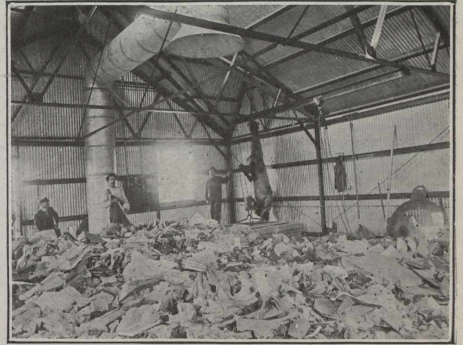
Fig. 2.—Dumping and Feeding Floor Showing Ventilating Airduct Leading to Pre-heater and Furnace.
