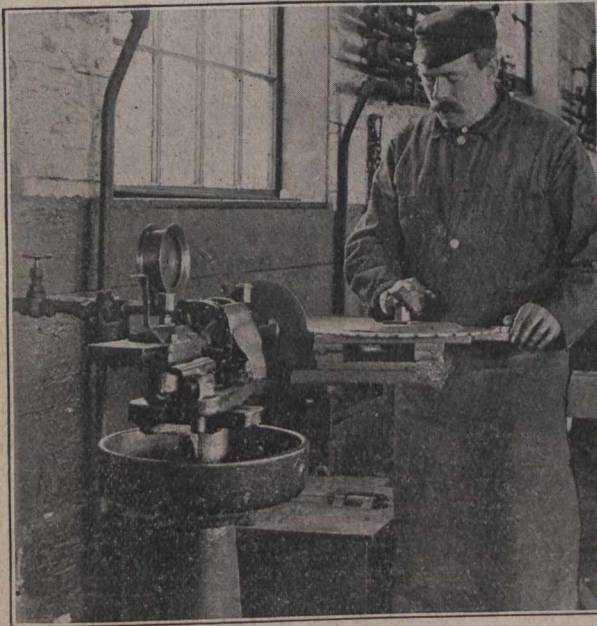
Air Motor Grinder for Sharpening Rail Saws.
