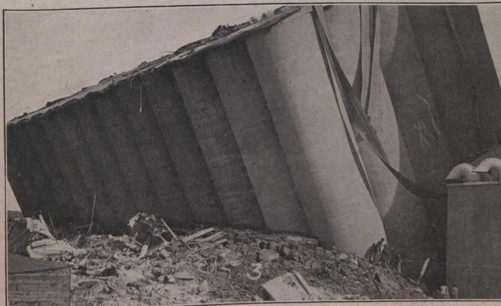
concrete bin house settled into the ground, by the crushing out of the foundation subsoil, and at the same time tilted to the posi-
