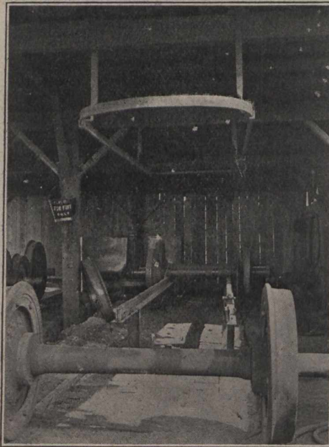
Tire Heating and Mounting Shed with Convenient Facilities.
