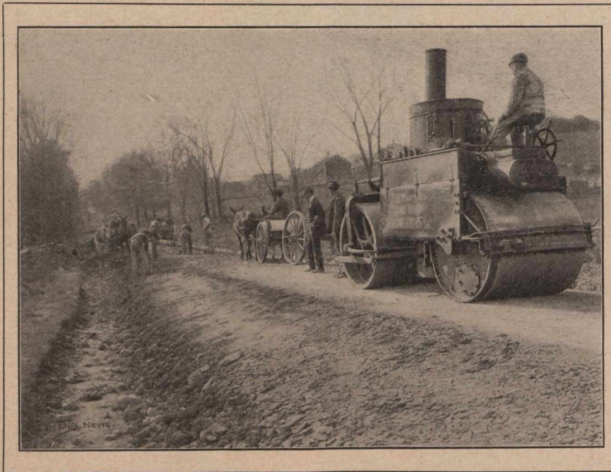
A STEAM ROAD ROLLER AT WORK.
