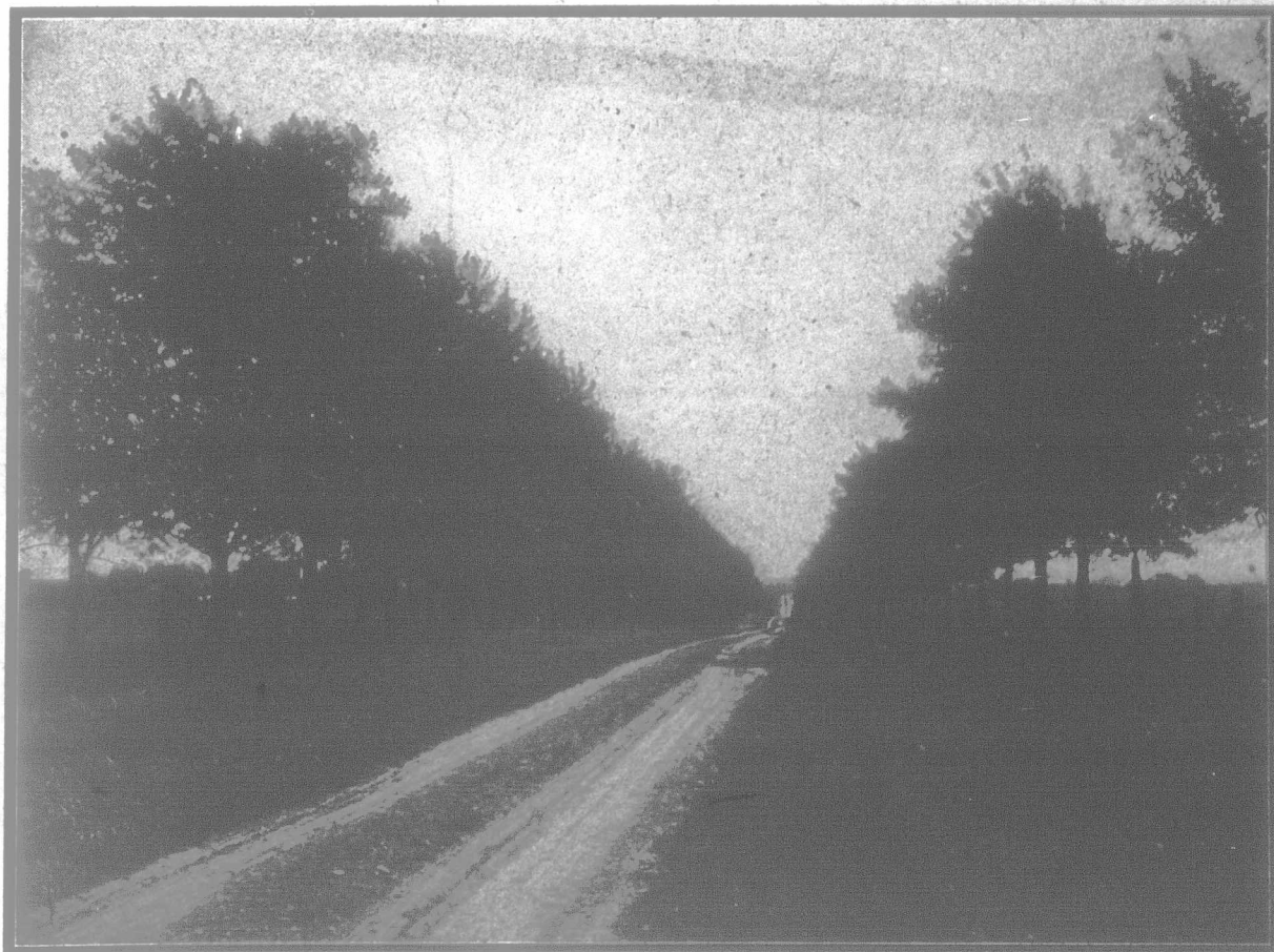
County Roads Well Rounded and Drained Stand the Test of Fall Rains.
