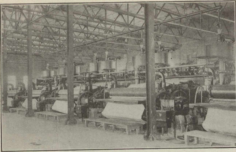
Wet machines, showing cylinder vat, felt, the roll on which the pulp winds up, and table for folding the "lap."
