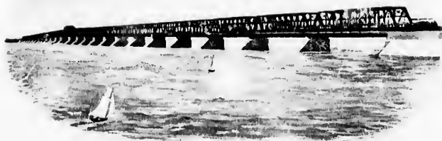
VICTORIA JUBILEE BRIDGE Opened for Traffic December, 13th, 1898
