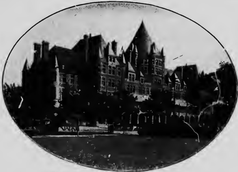
Canadian Pacific Railway Place Viger Station.
