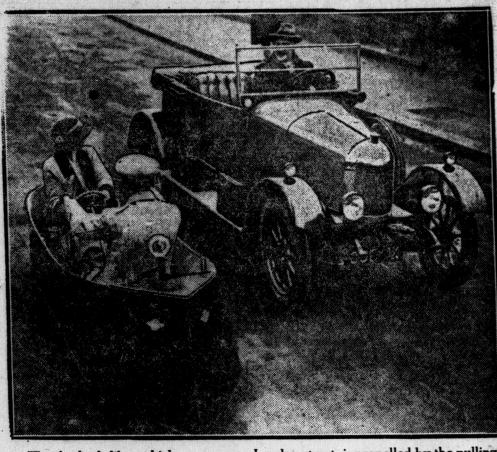
This bathtub-like vehicle, seen on a London street, is propelled by the pulling of two levers much as one pulls oars of a rowboat. The rider sitting in the back steers the craft
