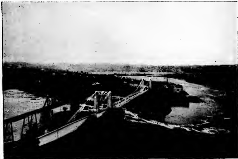
CANTILEVER AND SUSPENSION BRIDGES OVER FALLS, RIVER ST. JOHN.
