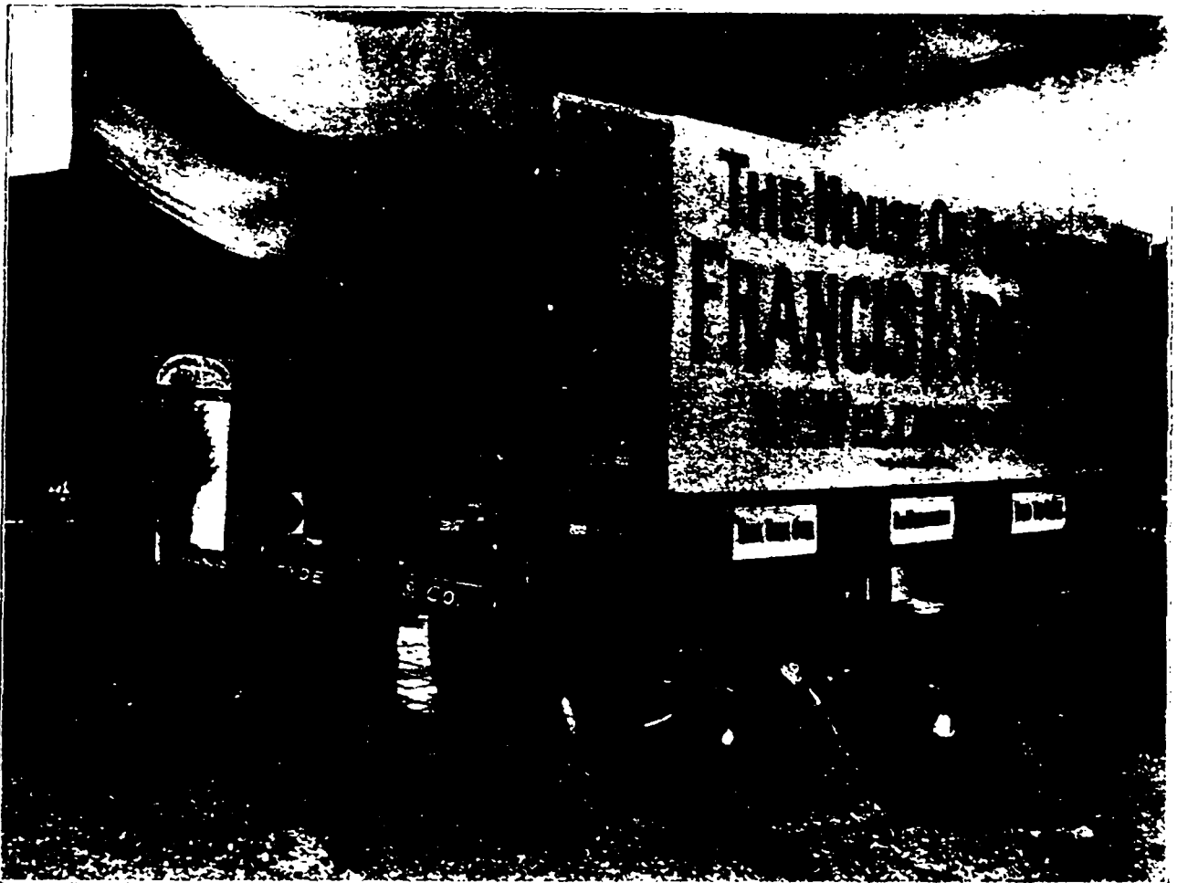
FRANCIS HYDE & CO., MONTREAL, AT THE MONTREAL BUILDERS' SHOW
