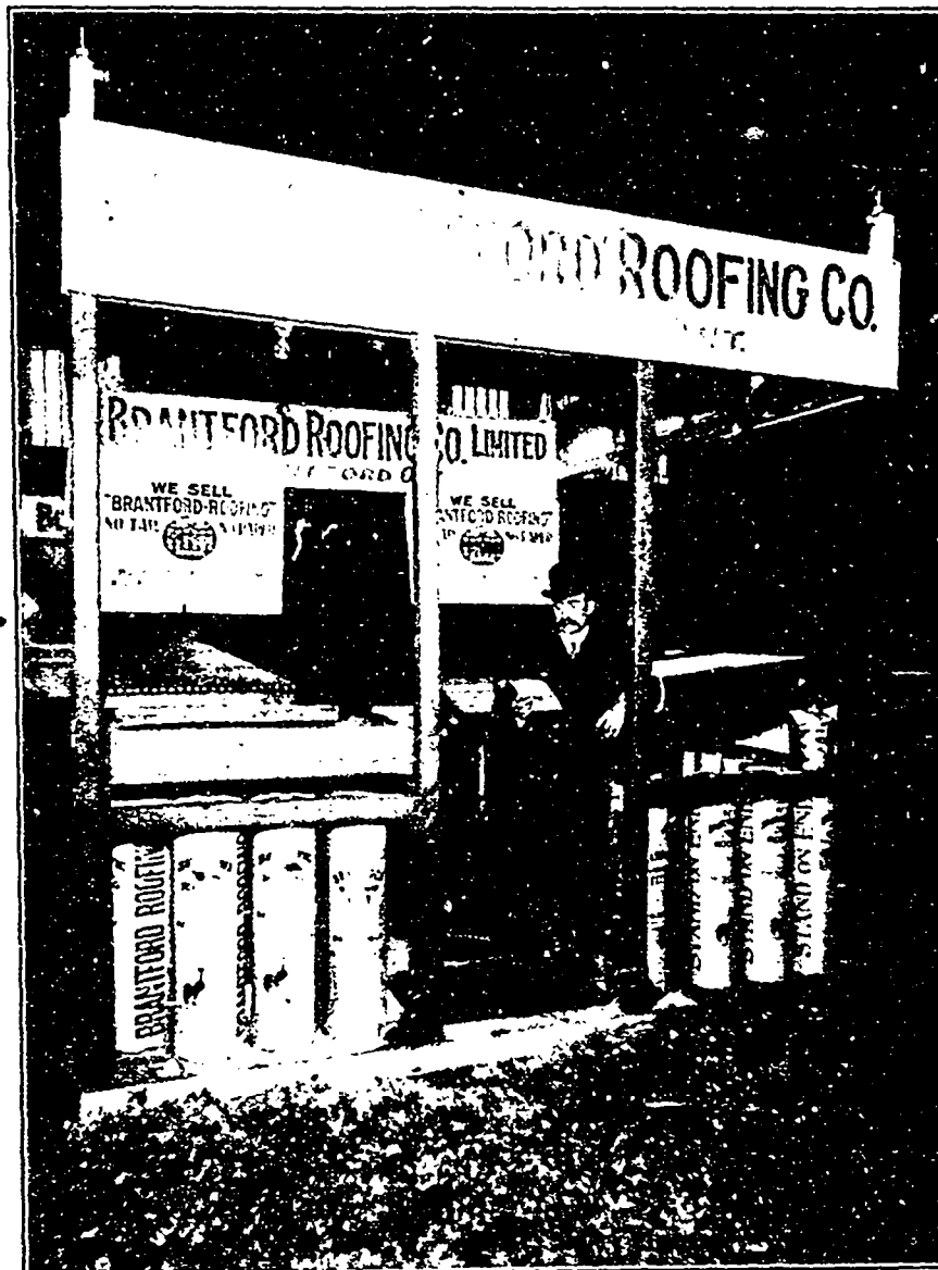
THE BRANTFORD ROOFING CO., BRANTFORD ONT., AT THE MONTREAL BUILDERS' SHOW
