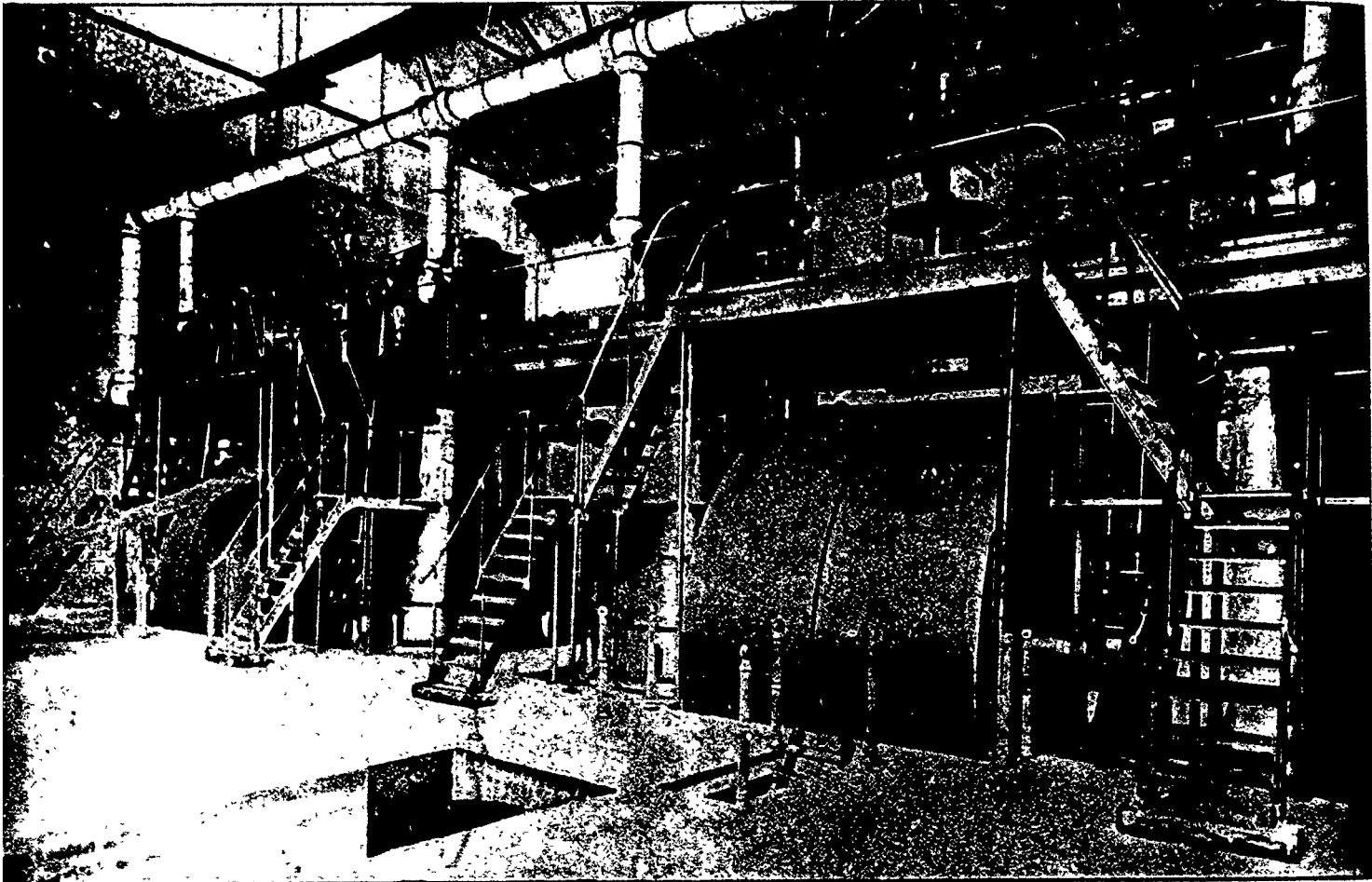
3,000 H.P. ENGINES IN No. 3 STATION, TORONTO ELECTRIC LIGHT CO.
