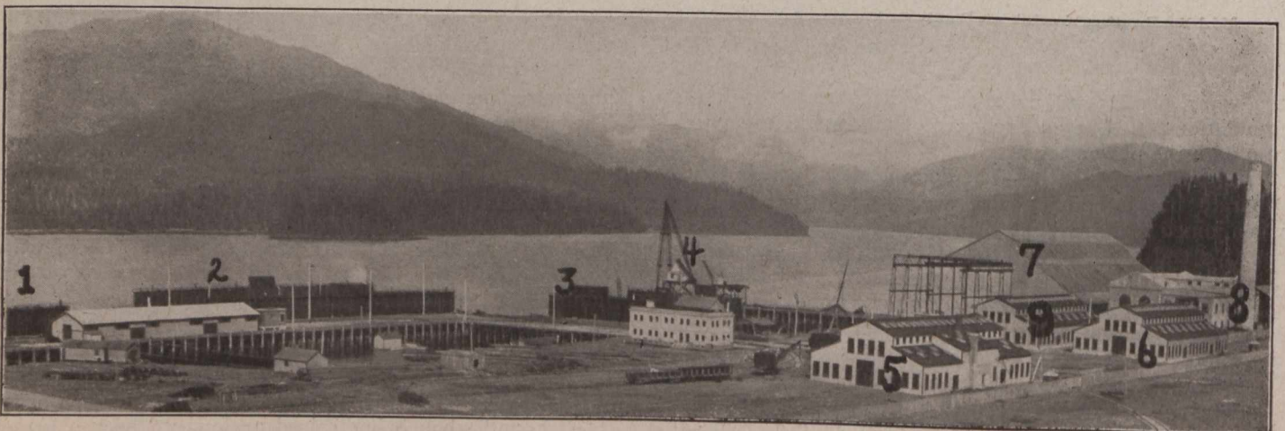
General View of Harbor and Terminal, Showing (1) End Section of Dry Dock, (2) Middle Section, (3) End Section, (4) Pier Derrick, (7) Shipbuilding Plant, (8) Power House, (5, 6 and 9) Foundry, Blacksmith and Boiler Shop, and Machine Shop.
