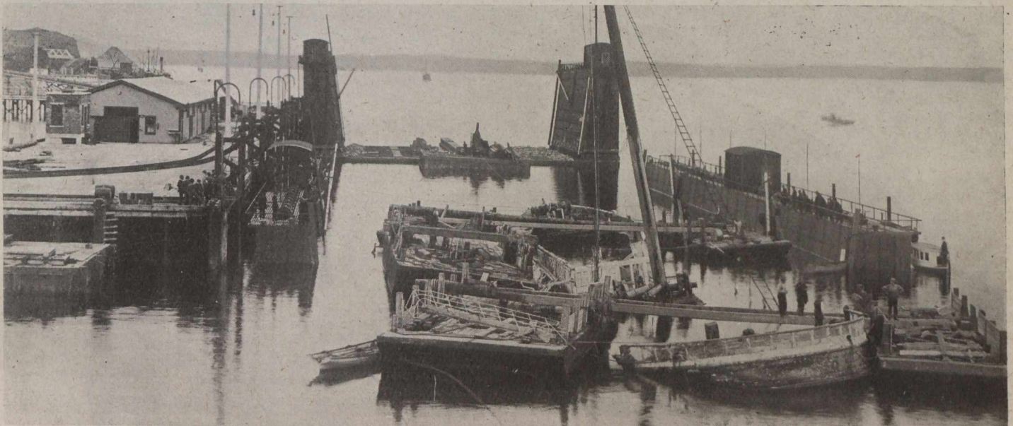
Middle Section (only) of Dock Submerged. Wrecked Vessel "Delhi" Being Lightered onto Submerged Section. One End Section, Not Submerged, in Background.
