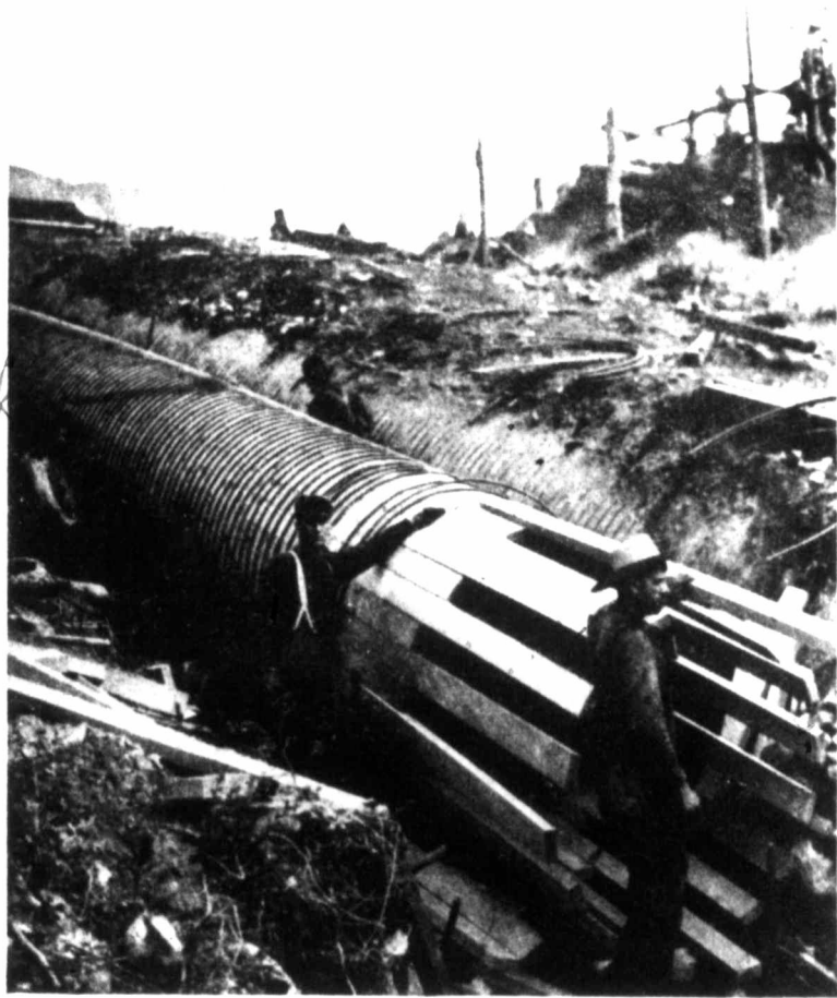
WOODEN STAVE PIPE LINE IN PROCESS OF CONSTRUCTION
