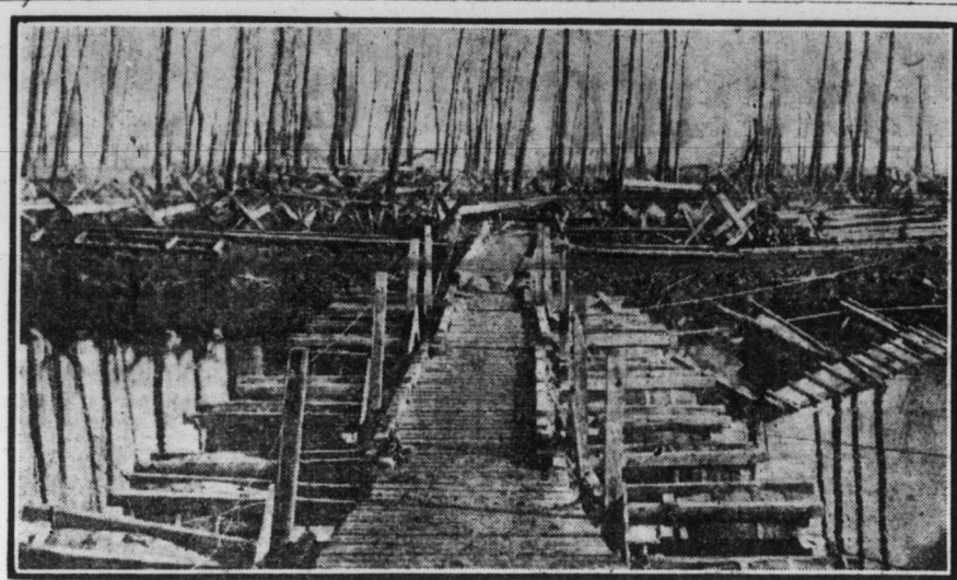
A British Cask-Pontoon Bridge Over the Yser, Constructed in One Night.
