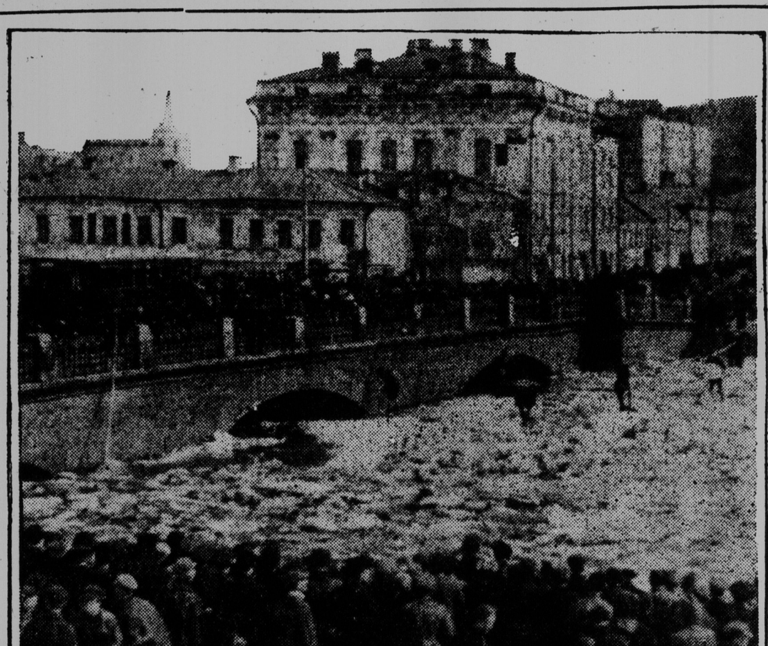
The Moskva river, flowing through Moscow under a score of bridges, has risen to such a height that its ice-filled waters have torn away several spans and threatened the larger ones. Photo shows one of the Moscow bridges with men working to break the ice blockade.
