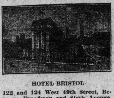
HOTEL BRISTOL 122 and 124 West 49th Street, Between Broadway and Sixth Avenue.
