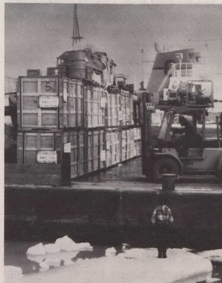
In mid-August, barges with prefabricated housing components are unloaded on the ice-rimmed shore of Holman Island.
