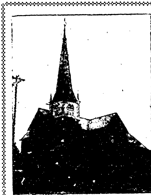
The New Queens Ave. Methodist Church. New Westminster.
