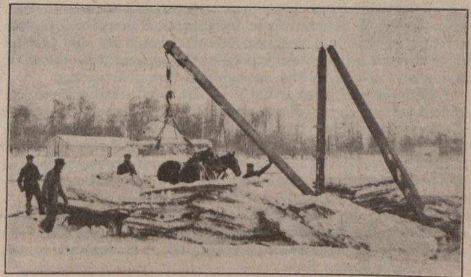
UNLOADING AND PILING SLABS AT POOL
