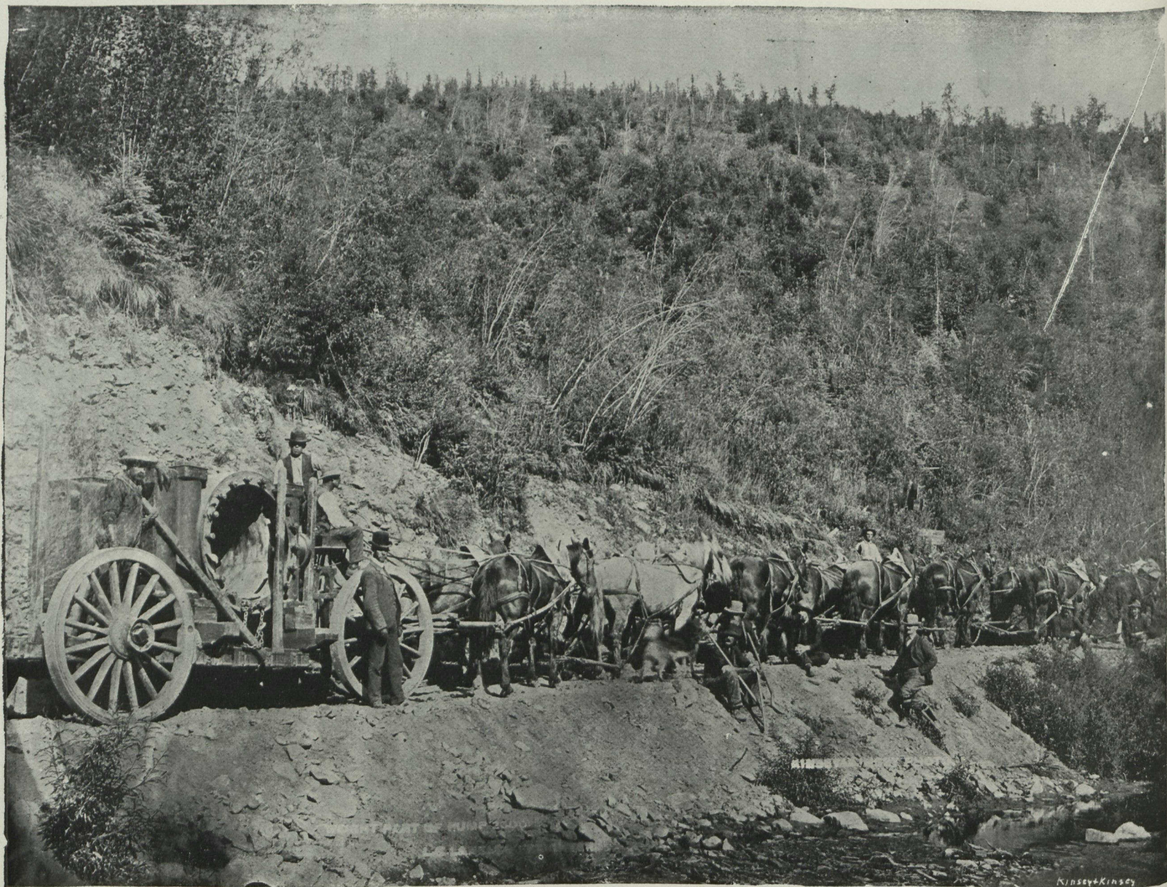
Cylinder head for Pacific Coast Mining Co.'s hydraulic plant on Bonanza, weight of load 26,000 pounds. Heaviest hauled in Klondike.
