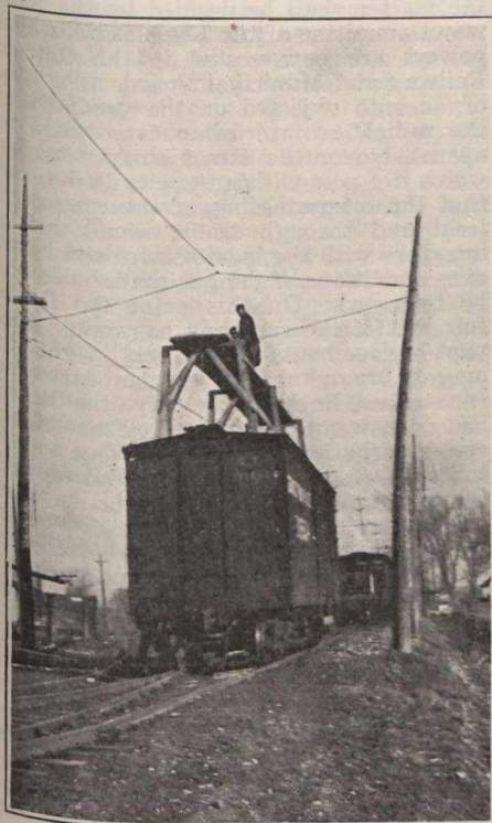
Stringing Overhead Work.
