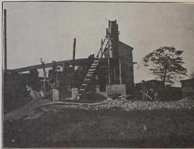
Colonial Coal Co.—Briquette Machine and Mixer.
