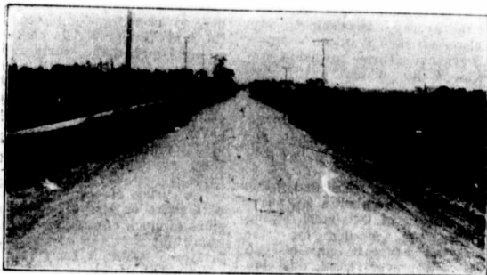
A Stone Road Built in Welland County.
