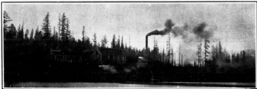
A General View of the Smelter.
