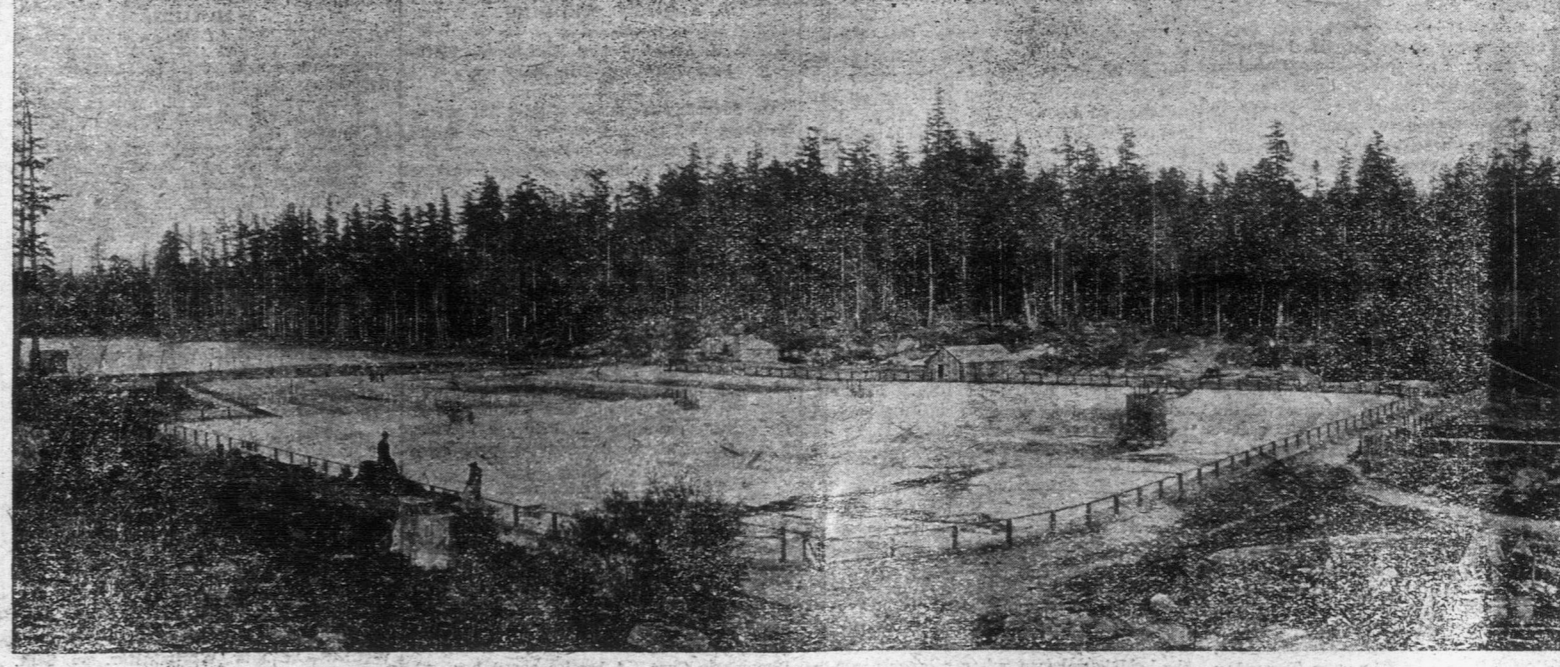
FILTER BEDS, BEAVER LAKE—FROM WHICH THE CITY DERIVES ITS PRESENT SUPPLY.
