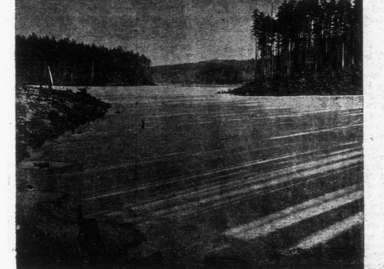
RESERVOIR AT GOLDSTREAM—NOW USED BY THE B. C. ELECTRIC RAILWAY COMPANY.
