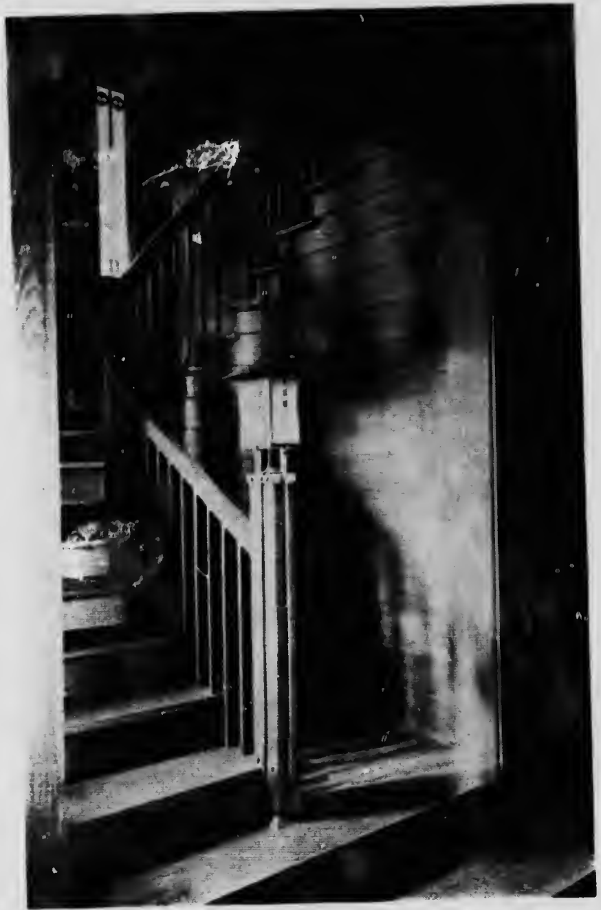
FIG. 89.—A good staircase well designed on conventional lines. The attention of the reader is directed to the rich effect obtained from the simple treatment of balusters and hand-rail.
