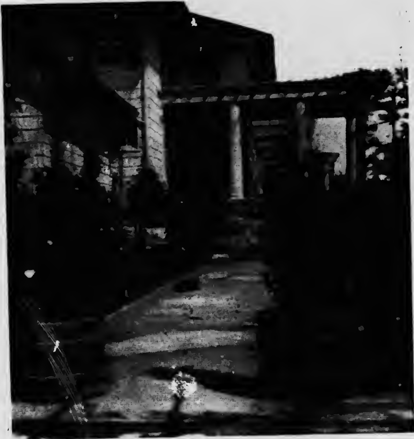
FIG. 46.—An old-fashioned treatment of the immediate surroundings of the house.
