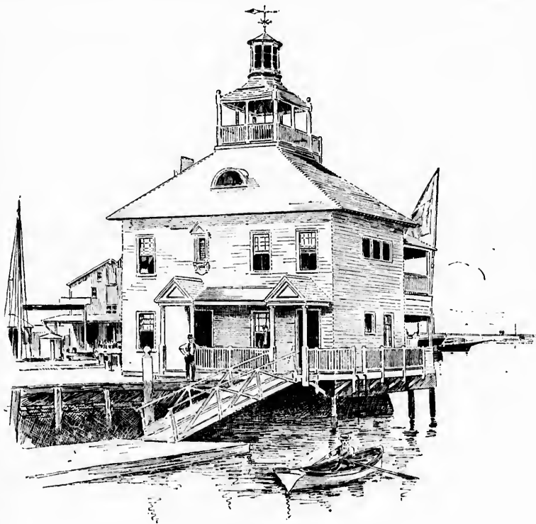
STATION No. 6: NEWPORT.—FIGURE 235.
