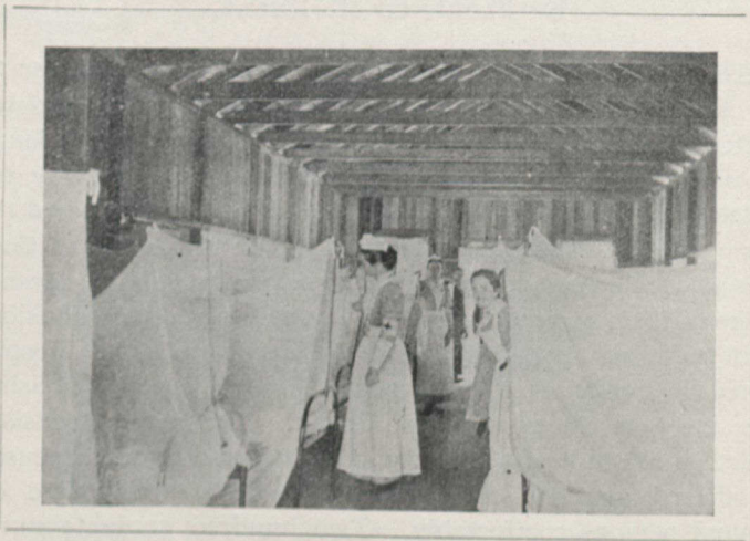
INTERIOR VIEW OF PAVILLION D.
