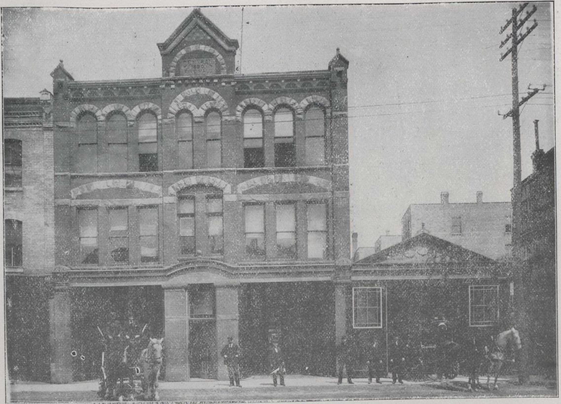
NO. 1 STATION FIRE HALL—LONDON.
