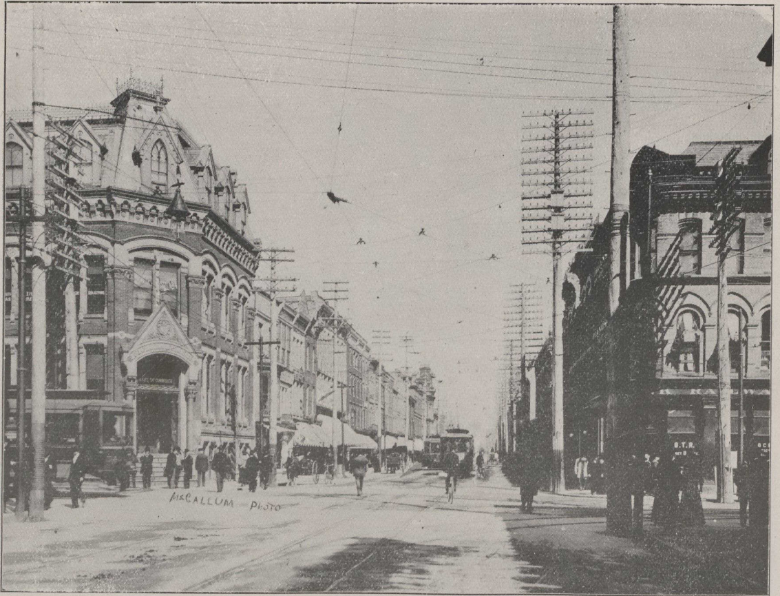
DUNDAS STREET, LOOKING EAST—LONDON.
