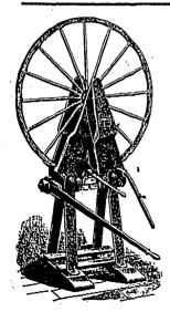
A truly wonderful and efficient machine for setting tires "cold" BY HAND without taking out the bolts.
