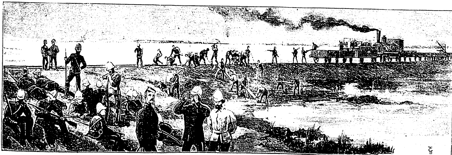
A WORKING PARTY REPAIRING THE CAIRO RAILWAY DESTROYED BY ARABI THE WAR IN EGYPT.—SKETCHES BY OFFICERS OF THE NAVY AND MARINES.
