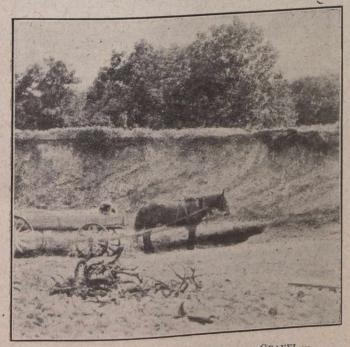
FIG. 4-LAKE ALLUVIAL DEPOSIT OF GRAVEL-NOTE STRATIFICATION
